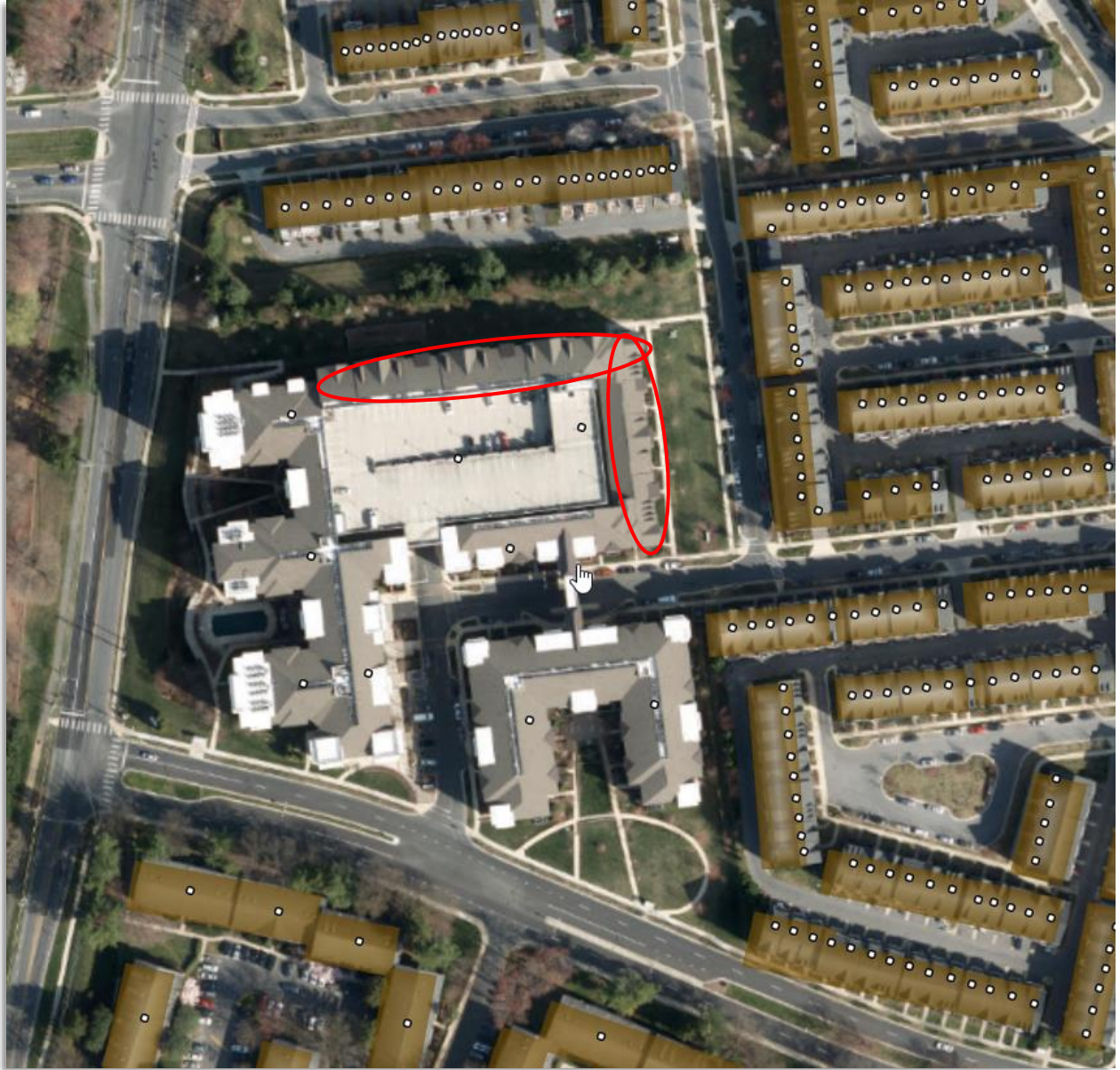
Figure 2: Missing Apartment Complex Structure
